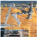
FIBERGLASS STRUCTURES AROUND WELLHEADS AND VESSELS
