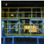
DRY TREE WORK PLATFORMS
