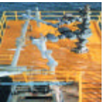
FIBERGLASS STRUCTURES AROUND WELLHEADS AND VESSELS
